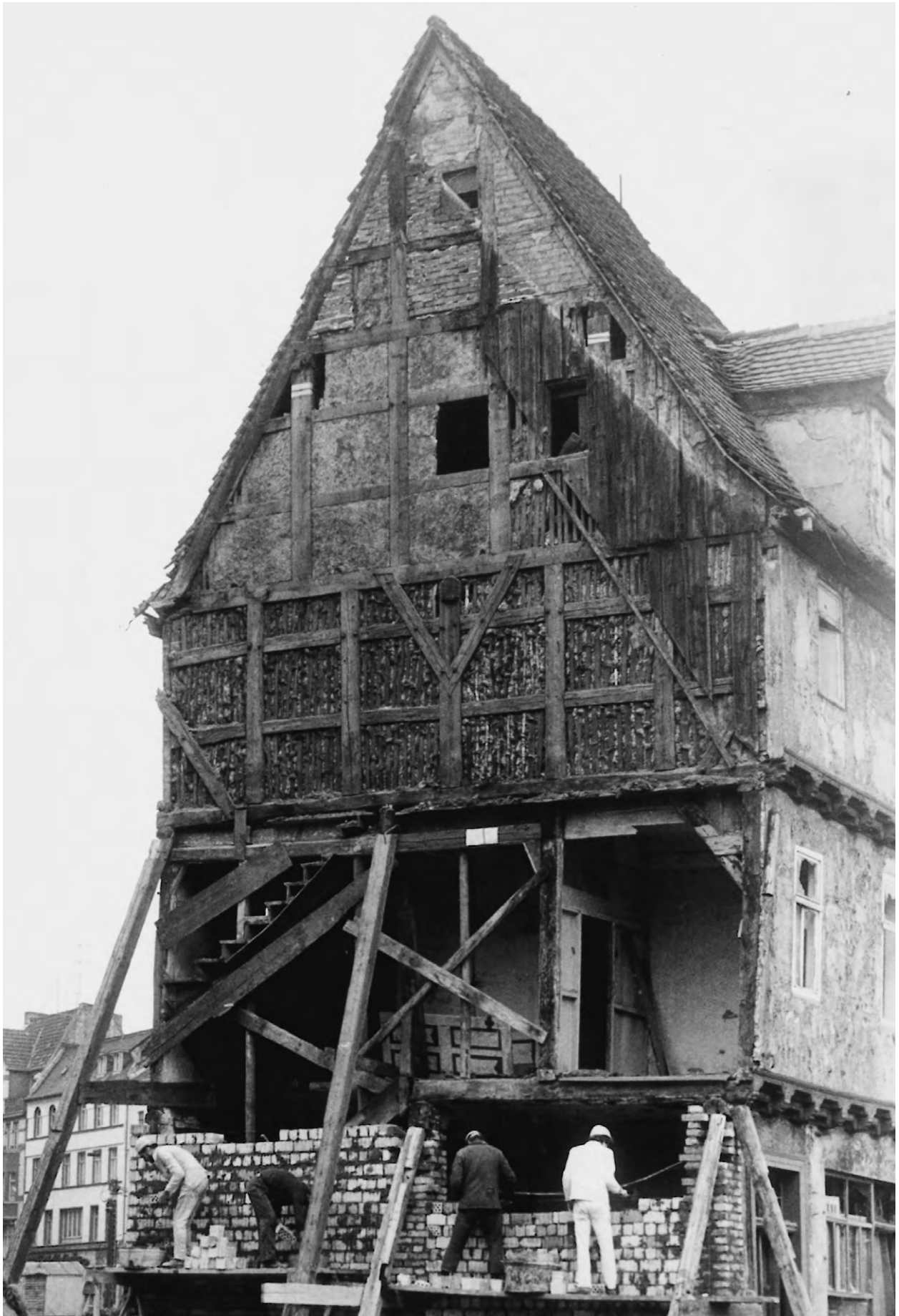
Securing the timber-framed house Alter Markt 31 in Halle (Saale), 1985
