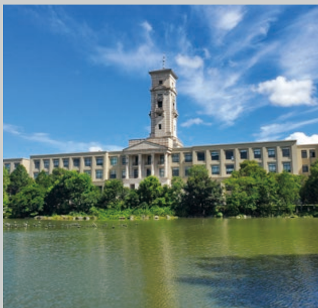
Trent Building in Ningbo
